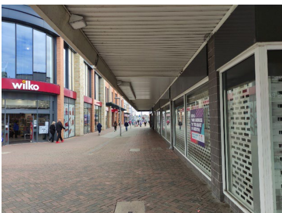
View under existing canopy
